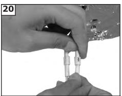
Connect white wire from fan to white wire from light fixture. Then plug black wire from fan to black wire from light fixture.
